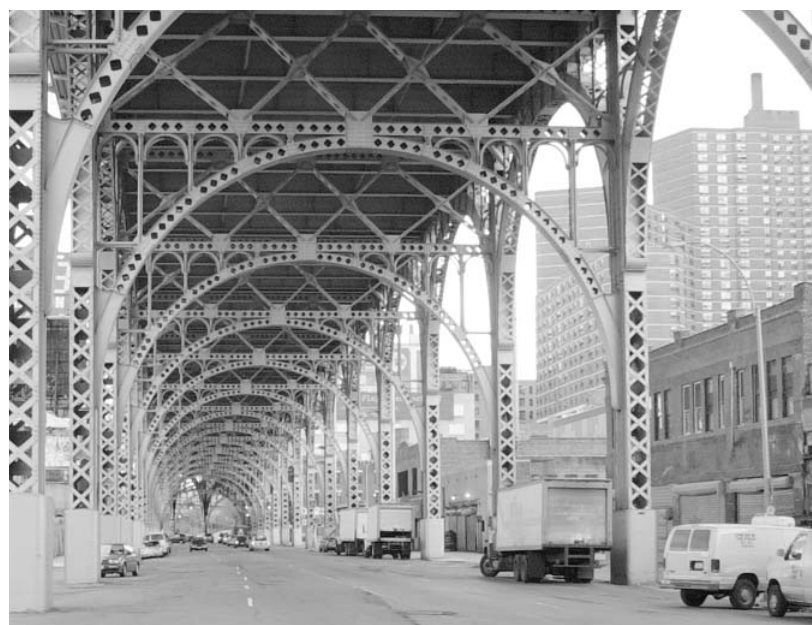
Viaduct near the historic Harlem Piers.
