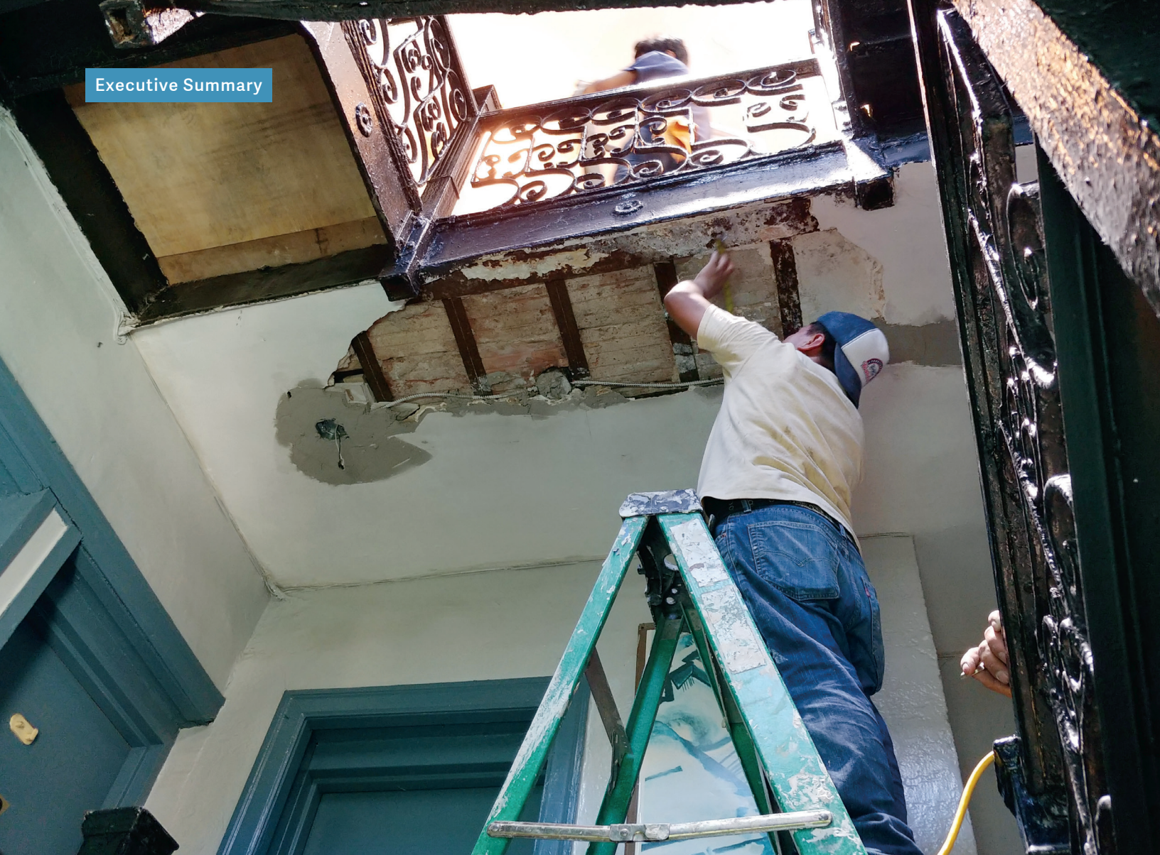
Workers disturbing old paint without protective materials or clothing at 332 East 4th Street © Evan Bell
